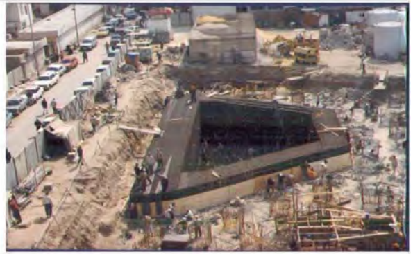
KAJIMA CORPORATION 870 Room Hotel at le Meridian Foundation Work (RE-BAR WORK).
