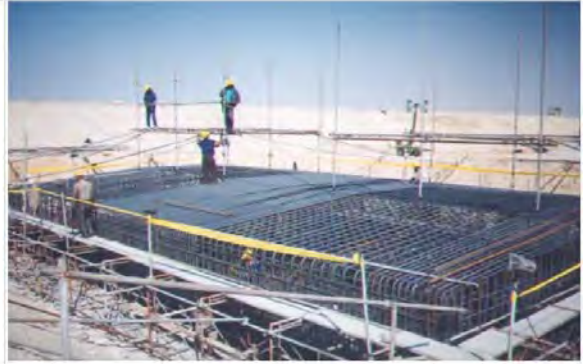
The Project Of Suez Canal Bridge Central Section In The Arab Republic Of Egypt (Kajima NKK-Nippon Consortium) Pile Cap Work.
