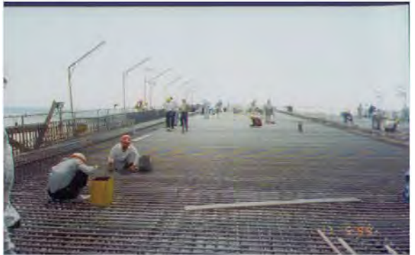
The Project Of Suez Canal Bridge Central Section In The Arab Republic Of Egypt (Kajima NKK-Nippon Consortium) Box Girder Work.
