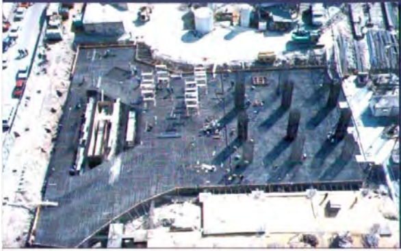
KAJIMA CORPORATION 870 Room Hotel at le Meridian Foundation Work (RE-BAR WORK).
