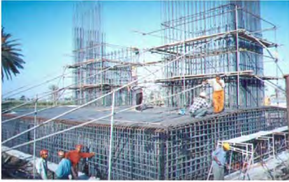
The Project Of Suez Canal Bridge Central Section In The Arab Republic Of Egypt (Kajima NKK-Nippon Consortium) Pile Cap Work.
